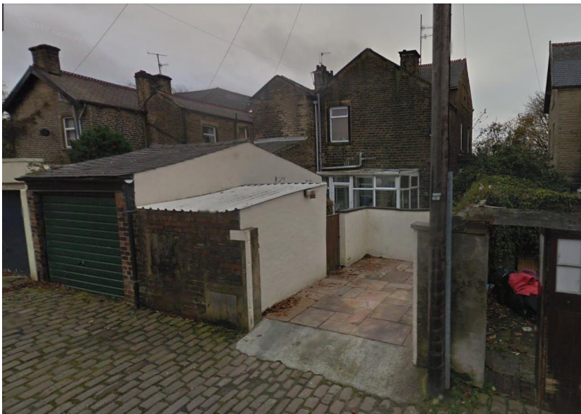
Photo 1: Rear of no. 4 Park Avenue (from Pendlehursts Street.) (Image taken from google street view)
